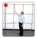
Add the mag bars onto the frame for front, D-ends and if applicable, the rear.
